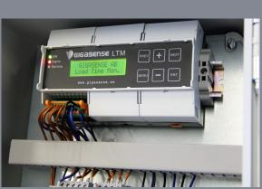
Gigasense LTM Load Time Measurement unit measures load hours.
